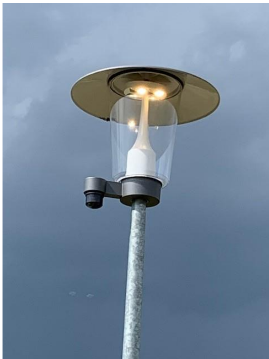
Figure 2: Luminaire with Zhaga-Interconnector
